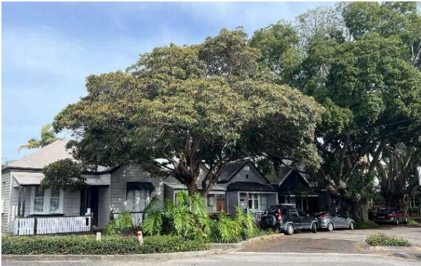
Figure E2.01: Street lined with mature trees alongside single-storey workers cottages contributing significantly to the streetscape.
