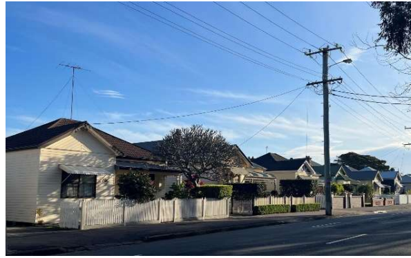
Figure E2.08: Array of federation cottages featuring the single-storey scale, uniform subdivision pattern, consistent street scape with front gardens, timber fence, and side driveways.
