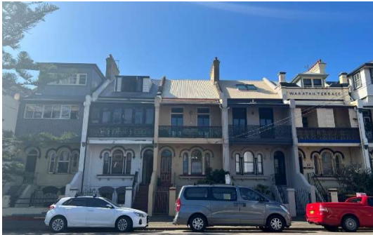
Figure E2.28: Row of three-storey terraces demonstrating the regular pattern of subdivision, ornate elements present in buildings constructed from mid-19 th and early 20 th centuries.
