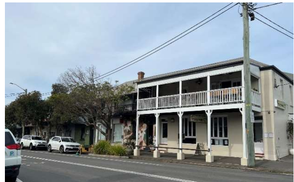
Figure E2.04: Cantilevered balconies with ornate elements over footpath in high street/commercial premises.
