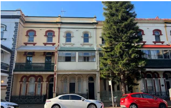
Figure E2.32: Row of three storey terraces with uniform urban form, ornate elements contributing significantly to the historic character of The Hill.
