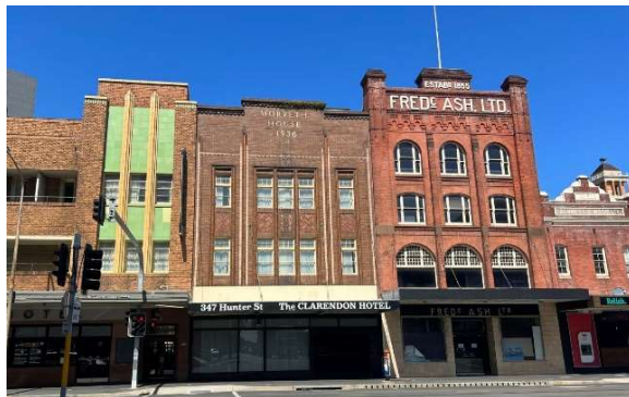
Figure E2.24: Buildings built in mid-19 th to early 20 th centuries enhance the rich historic character.
