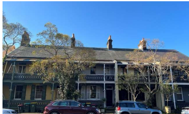
Figure E2.33: Two-storey housing stock - the original defining feature of the area, complemented by street trees.
