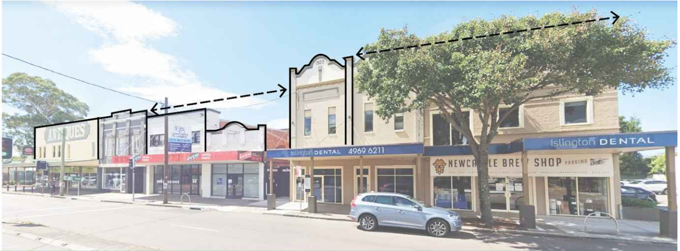
Figure E8.36: Existing parapets dominating the street edge
