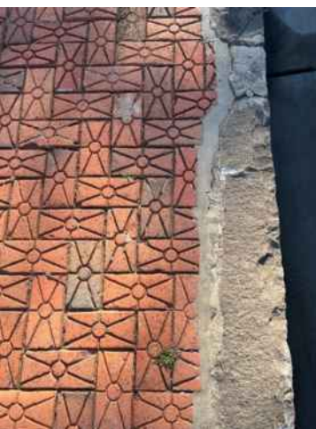
Figure E2.34: Heritage road assets such as sandstone kerbing and restored historic pavements.
