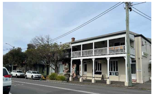
Figure E2.04: Cantilevered balconies with ornate elements over footpath in high street/commercial premises.
