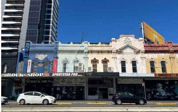
Figure E2.22: Row of buildings with consistent urban form, design elements and fine grain.
