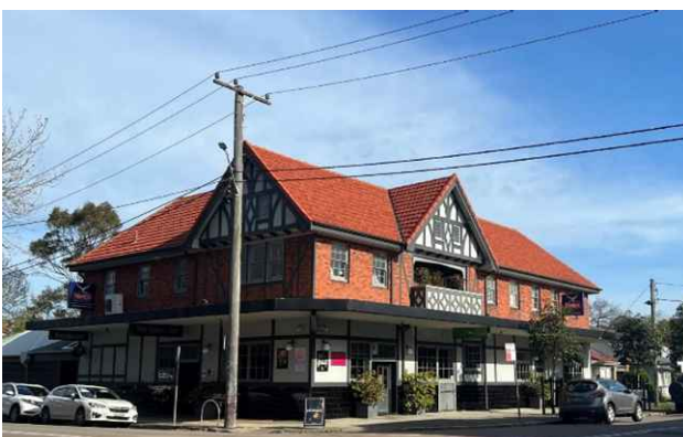
Figure E2.05: Heritage building with commercial use.
