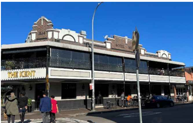
Figure E2.12: Contributory building constructed prior to second world war with cantilevered cast iron balconies adorned with decorative lacework over the footpath on Beaumont Street.
