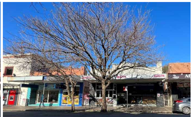
Figure E2.13: Mix of single and two-storey buildings consisting of uniform subdivision pattern, active frontages with sandstone kerbing and trees present in public domain.
