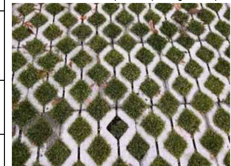
Figure C4.03: Porous Paving Example
