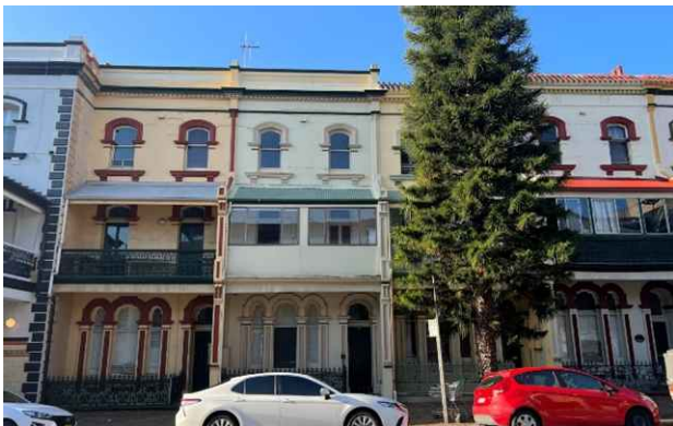
Figure E2.32: Row of three storey terraces with uniform urban form, ornate elements contributing significantly to the historic character of The Hill.
