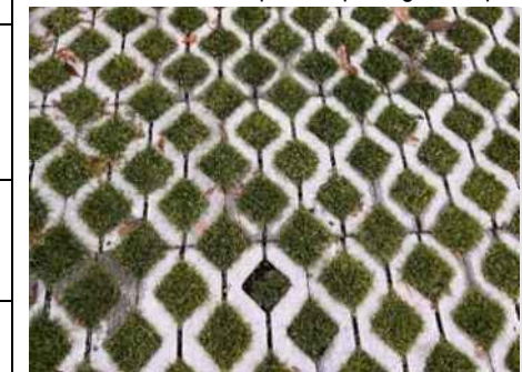
Figure C4.03: Porous Paving Example
