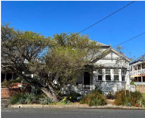
Figure E2.16: Cottage with original ornate elements, mature trees in the public domain with sandstone kerbing contributing to historic character.
