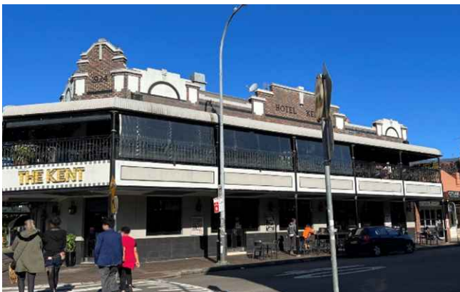
Figure E2.12: Contributory building constructed prior to second world war with cantilevered cast iron balconies adorned with decorative lacework over the footpath on Beaumont Street.
