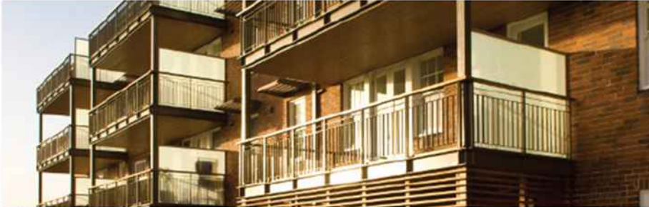
Timber coastal apartments - Wood Solutions
