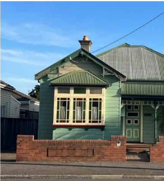
Figure E2.09: Federation cottage exhibits original design elements of federation style.
