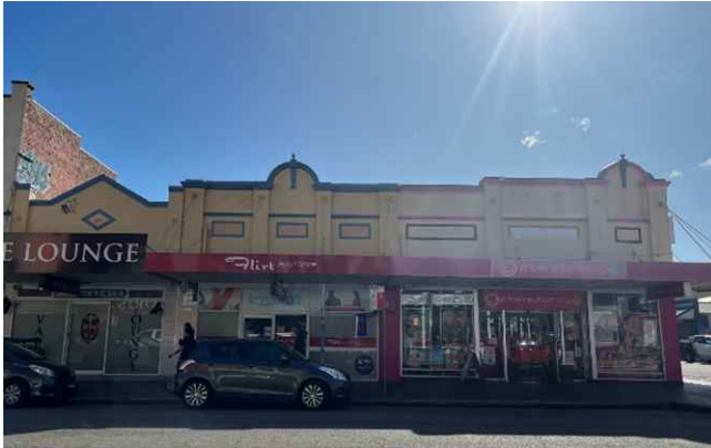
Figure E2.10: Commercial buildings with active frontages and parapet wall concealing the roofs.
